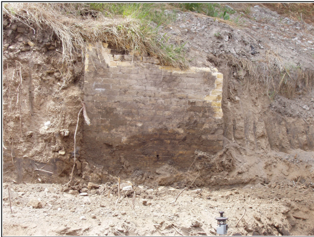
Figure 4-17. Feature 6, yellow brick wall (see Figures 4-1 and 4-12).
