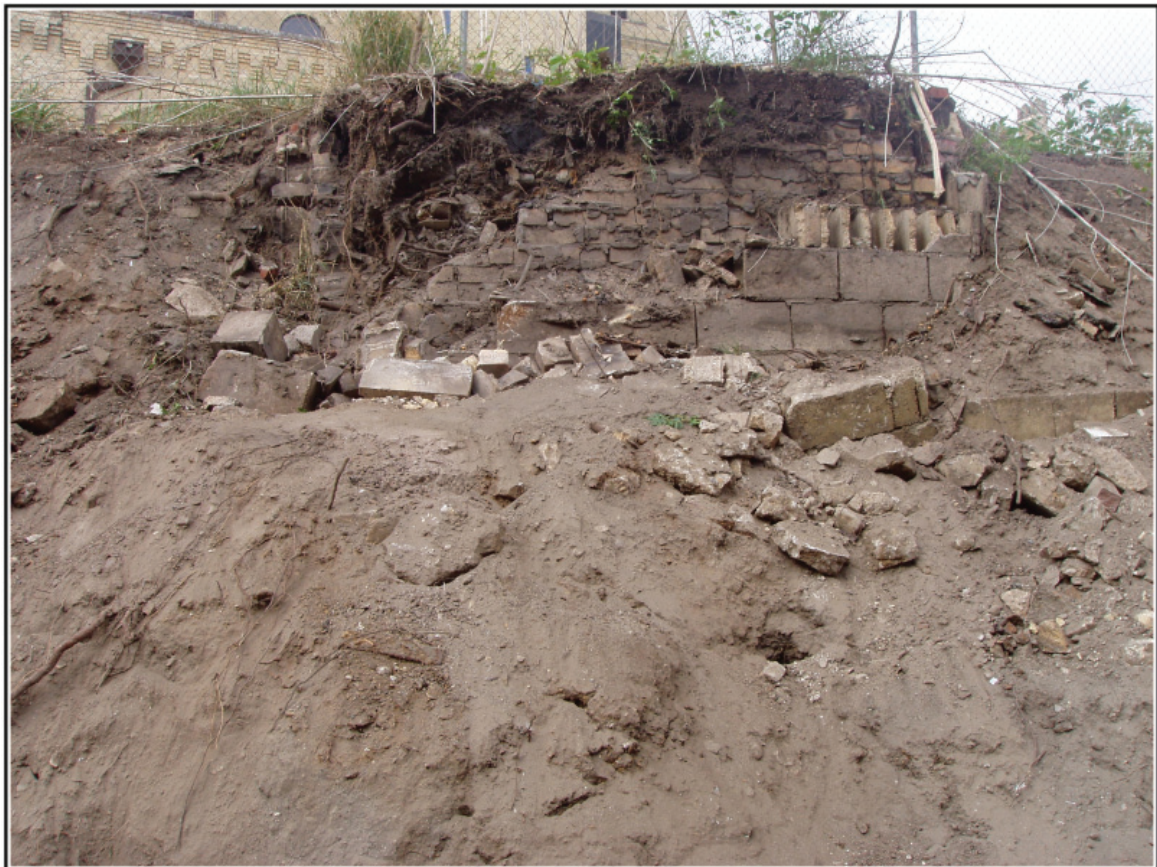
Figure 4-16. Feature 5, brick wall (see Figures 4-1 and 4-12).
